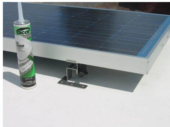
The attachment points need sealing with a good adhesive.
