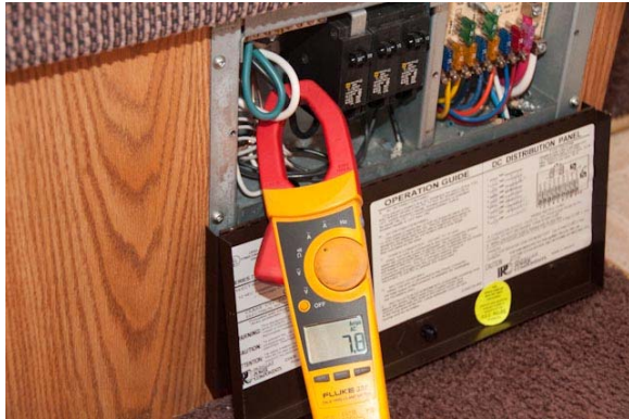
The clamp can be used on any breaker in the box
