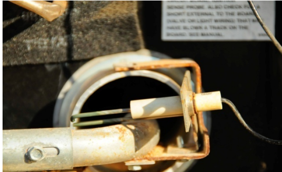
Check for cracks in the porcelain on the electrode
