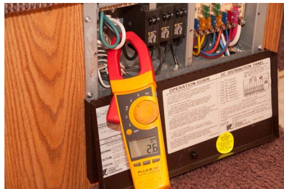
Measuring amperage through the main breaker at the distribution panel
