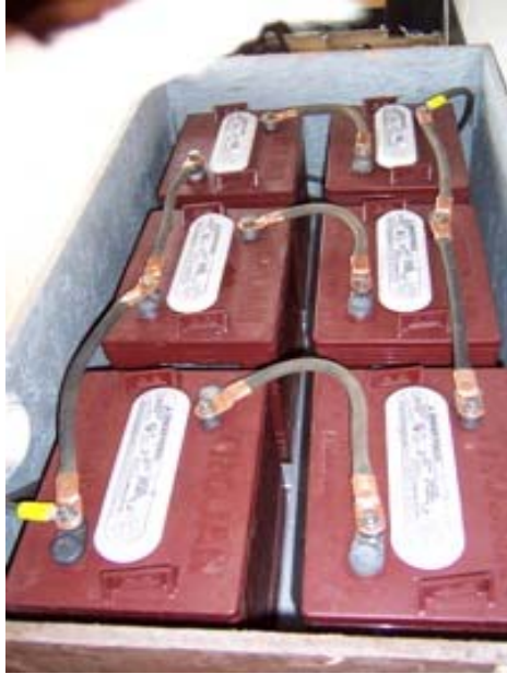
Battery cells can be drained by small loads like clocks and control panel indicators.
